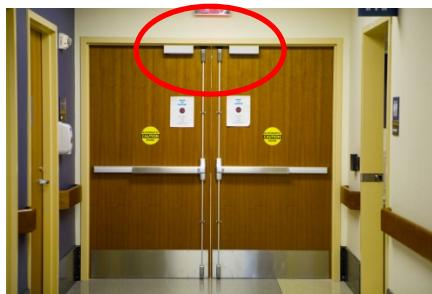
Mag lock doors basically have 2 locks – the magnetic lock plus the actual door hardware lock. Please keep the following in mind for mag lock doors –
